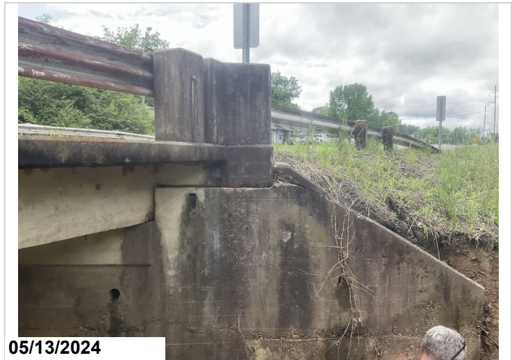
Abutment # 1, left: the wing wall is spalled adjacent to the end post.
