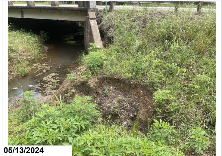
Abutment # 1, left: minor erosion adjacent to the wing wall and behind the wing wall.
