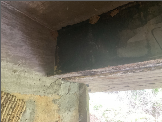
Abutment # 1, beam # 1: section loss to the beam end.
