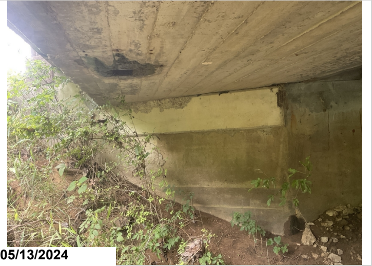
Abutment # 1, cap, right: the cap has spalling in the bearing area of the concrete slab.
