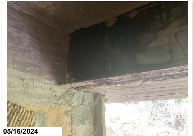
Abutment # 1, beam # 1: section loss to the beam end.
