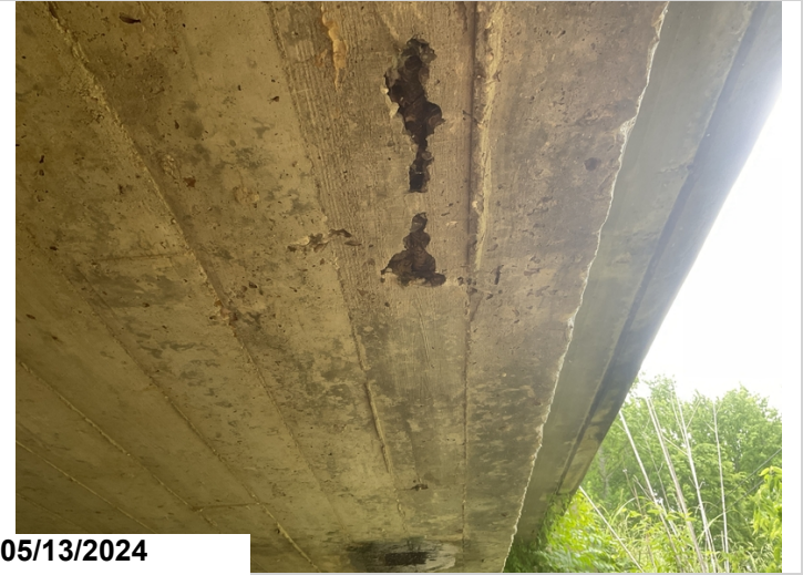
RC Slab Span, right: the exterior edge of the deck near mid span has a 12" long area of honeycombing with exposed reinforcing steel with no apparent section loss. Exposed reinforcing steel with no apparent section loss is visible in all 4 deck drains.
